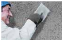
Cement-based render with MapeLatex 水泥基打底涂层 MapeLatex
