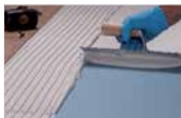
Stone material installation after 4 hours 四小时后可进行铺砖
