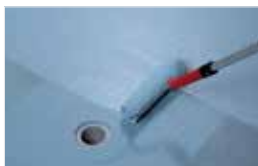
2nd coat after one hour 一小时后施涂第二层涂漆
