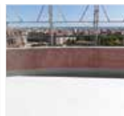
Completed with two top coats 两层涂漆即完成
