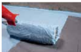
1st coat on existing tiles 第一层涂漆于瓷砖上
