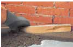
Application of a cement-based bonded screed admixed with MapeLatex 水泥基找平砂浆与 MapeLatex 混合使用
