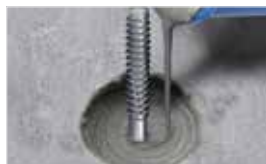
Anchoring of starter bars 锚固预留搭接钢筋
