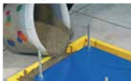
Filling gaps under baseplates 填充基座下的缝隙
