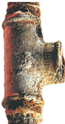
External corrosion - Steel
